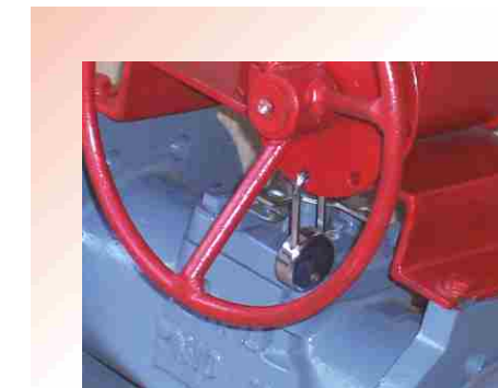
Gear with locking provision
